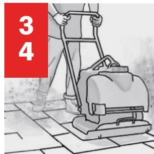
**3** Vibrate the GATOR POLYMERIC SAND into the paver joints using a vibratory plate compactor. A rubber pad is recommended. A roller compactor is best for slab installation.
