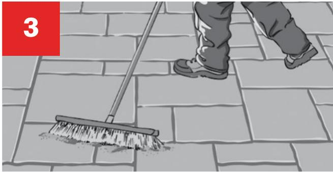
Sweep off excess SUPERSAND G2 from the paved surface, first with a hard-bristle broom, then a soft-bristle broom. Take care to leave the height of SUPERSAND G2 at least 1/8 inch (3 mm) below top of paver's surface or 1/8 inch (3 mm) below the chamfer.
