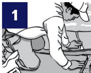
**1** Spread EUROSTONE BOND with hard-bristle broom. Make sure the EUROSTONE BOND completely fills the joints. Do not use with other materials in the joints. Leave a layer of EUROSTONE BOND on the surface to aid in the vibrating and consolidation of EUROSTONE BOND into joints.
