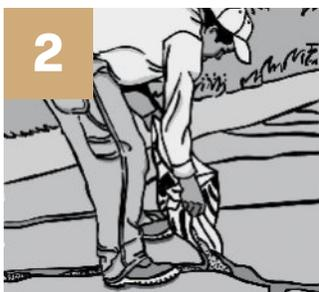
**2** Make sure the wet cast or natural stone top and side surfaces are dry.
