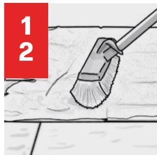
**1** Spread GATOR POLYMERIC SAND with a hard-bristle broom. Make sure the GATOR POLYMERIC SAND completely fills the joints. Do not use other materials in the joints.
