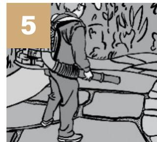
**5** Using a leaf blower, blow all GATOR DUST residues off wet cast or natural stone surfaces.
