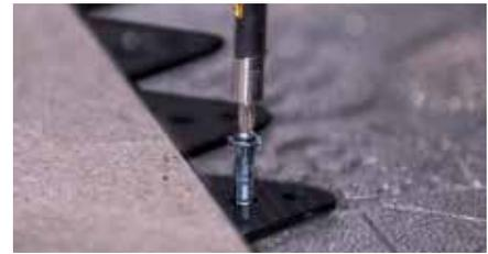
When using any of the Gator Edging on the Gator Base they must be fastened with Gator Base Screws only.
