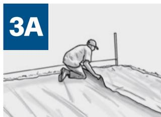
**A** Lay down the Gator Fabric GF 4.4 and cover the complete excavated area and sides.
