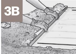
**B** Spread an even layer of sand, no more than 3/4" thick (19 mm) • Levelling and compacting the sand will be the last step prior to installing the Gator Base.
