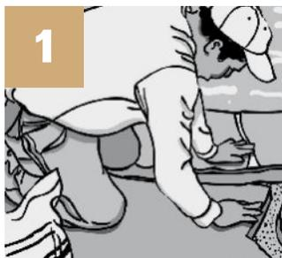
**1** Install the wet cast or natural stones on a maximum 1" (25 mm) bed of sand. Make sure that there is at least 6" (15 cm) of compacted crushed stone under the bedding sand. See diagrams below.
