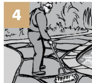
**4** Using a soft, fine-bristle broom, sweep all excess GATOR DUST off wet cast or natural stone surfaces. Ensure that GATOR DUST lies at least 1/8" (3 mm) below the top of the wet cast or natural stones or erosion may occur.
