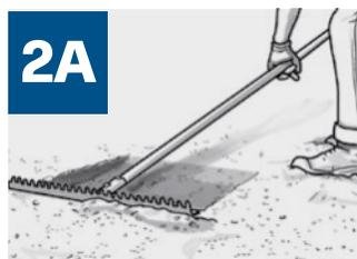
**A** Once excavation is completed, level the excavated area using a rake or shovel. Ensure a slope of at least 1 degree away from any structure, such as a house.
