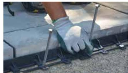
Alliance Gator Nails are high quality nails which are available in lengths of 10" (25 cm) and 12" (30 cm), common or spiral models. Gator Nails are designed for use with all Gator Edge types.
