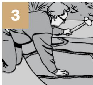
**3** Hit the wet cast or natural stones with a rubber mallet; this will make the GATOR DUST settle firmly into the joints by removing any air pockets. Repeat step 2 and this step 3 at least two more times.
