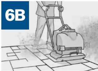
**B** Vibrate the GATOR MAXX **G2** into the paver joints using a vibratory plate compactor. A rubber pad is recommended. A roller compactor is best for slab installation. Joints should be filled up to 1/8" (3 mm) below the top of the stone or 1/8" (3 mm) below the chamfer. It is best to compact in several directions to ensure there are no air gaps or voids in the joints. Repeat steps 1 and 2 to ensure joints are filled and consolidated. Narrow joints require more care to completely fill.
