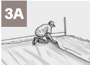
**A** Lay down Gator Fabric GF 4.4, a non-woven geotextile (minimum 100 LBF) and cover the entire excavated and compacted area.
